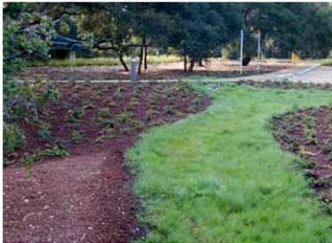
Site drainage and stormwater control systems employ bio-swales, detention ponds, and filtration devices to limit disruption of natural water flows, increase on-site infiltration, and eliminate contaminants. These measures help protect the ecology of the site, the surrounding neighborhood, and San Francisco Bay. Drought-tolerant landscaping featuring native vegetation combine to reduce water consumption by a projected fifty percent compared to similar, conventionally landscaped sites. Waterless
